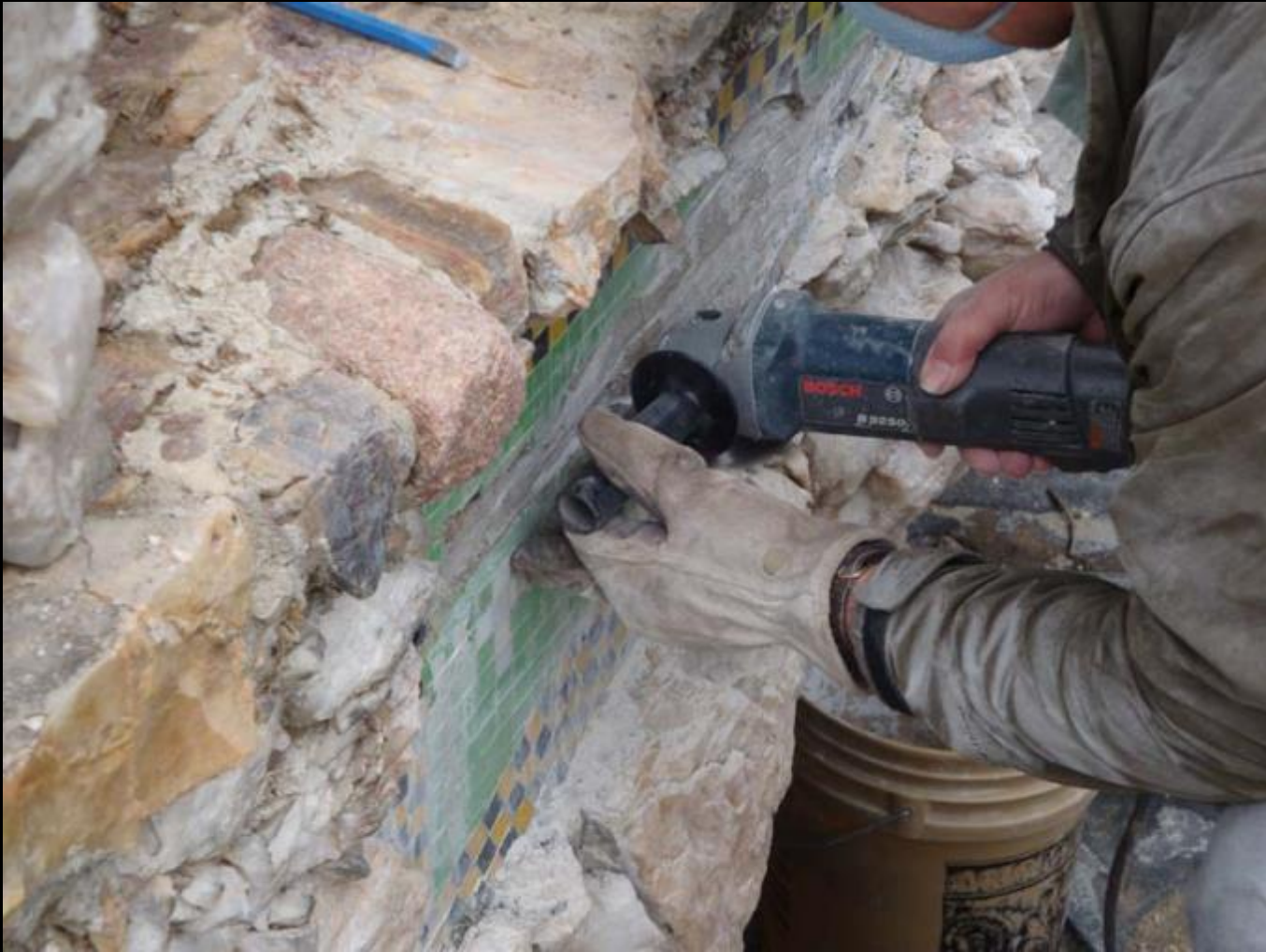
Gently grinding down old mortar
