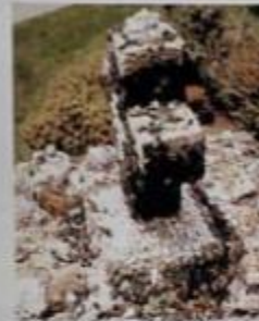
6. Loose black stones on left have become detached from top of cross.
